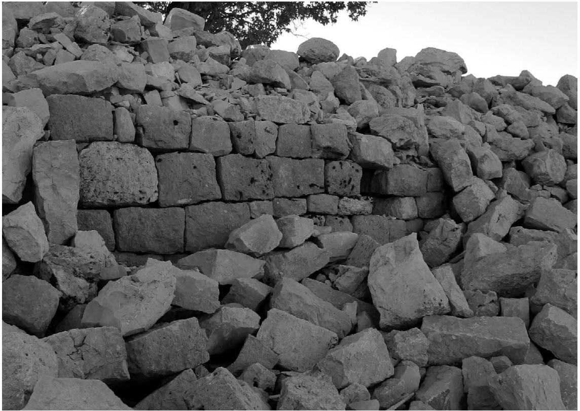
Fig. 41. Bilevah. Collapsed wall in stone blocks of masonry (Picture by J. Mehr Kian).
